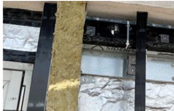
A photo showing Phase 1 South Elevation – Siderise cavity fire barriers installation works progressing.
